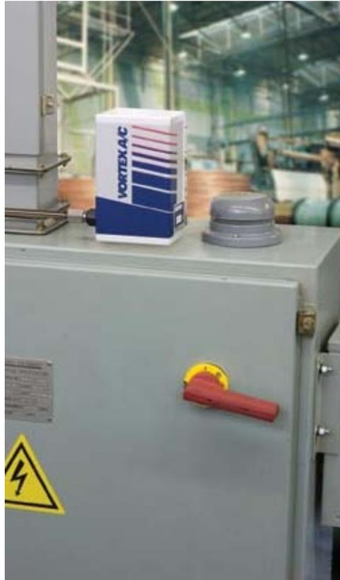
**The Vortex A/C meets NEMA standards for Type 4 and 4X rated enclosures, with models available to deliver 900, 1500, and 2500 BTUH of refrigeration.**
